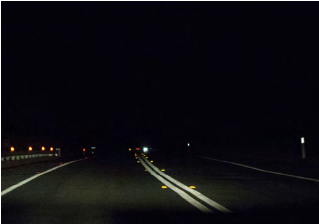
Figure 9. Wet Reflective Pavement Markings
