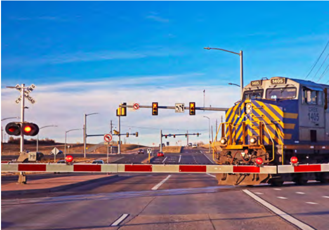
Figure 29. Active Railroad Warning Devices
