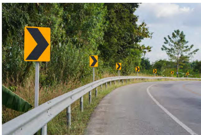
Figure 3. Enhanced Delineation for Horizontal Curves
