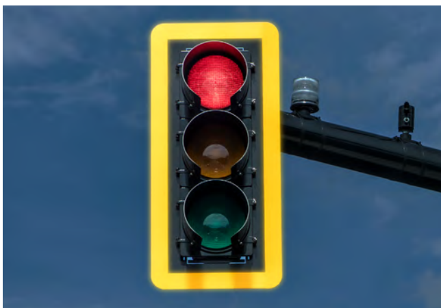
Figure 8. Retroreflective Backplates
