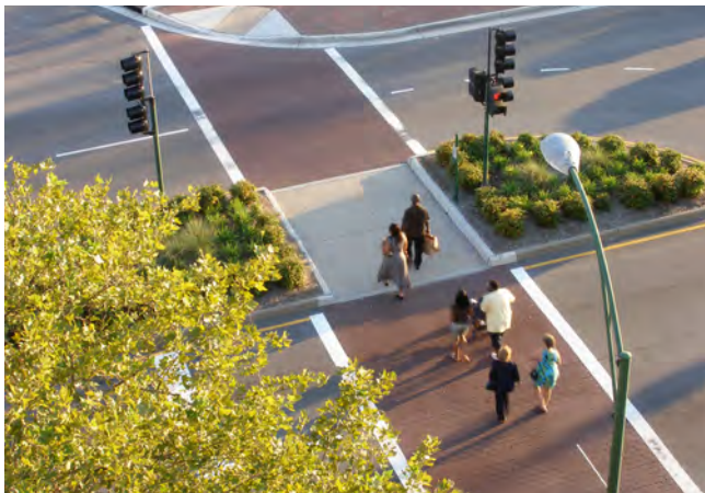
Figure 17. Median and Pedestrian Refuge Island
